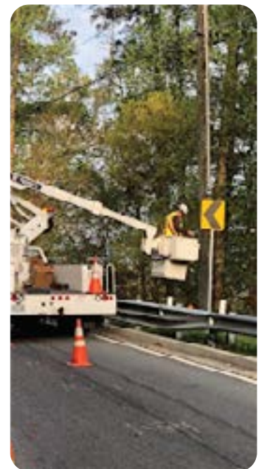
City Foot Traffic Street Electric & existing pole
