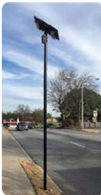
Entrance to Hotel Solar & Flock 14 foot pole
