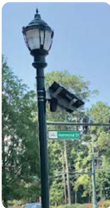
City intersection Solar & existing pole
