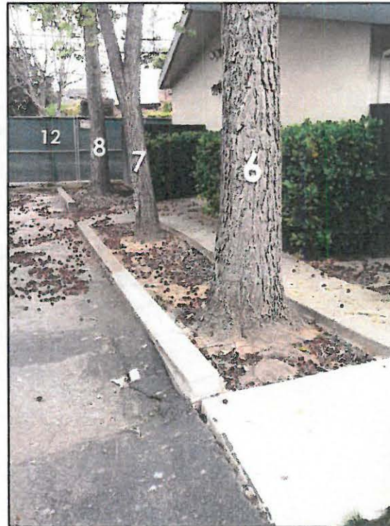
Close-up of pavement damage caused by the roots of sweet gums #6, 7 and 8.
