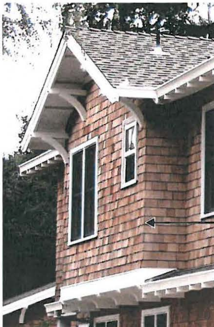
Mitered shingle corners
