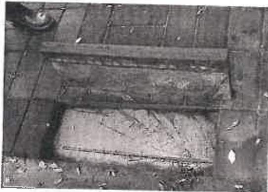
Figure 37. Recycled rubber is being tested as an alternative to concrete (A). Individual pavers or modules can be removed to inspect and treat underlying roots (B).
