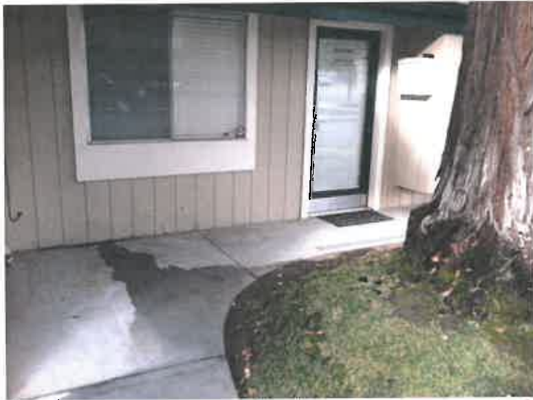
2014 – sloping concrete caused by tree forces water toward suite 105 and not away from the building resulting in water damage
