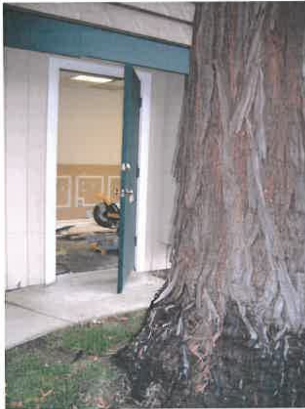
2007 Picture of Tree at Suite 105 obstructing the door opening because of raised concrete walkway.
