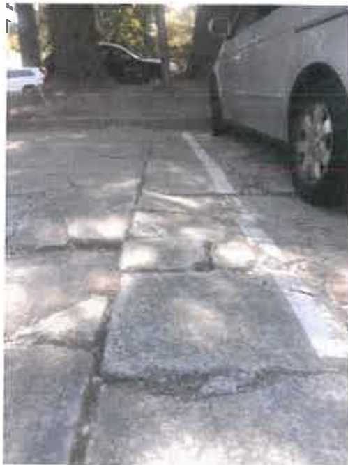
2015 – Picture of rear parking lot area and resulting damage caused by coastal redwood. This picture demonstrates that tree roots will break concrete. Fortunately the roots can be trimmed and concrete re-poured.
