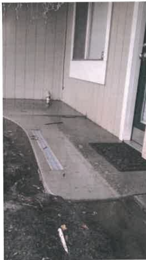
2014 – with more rain the drainage problem gets worse driving more water toward the building causing severe water damage
