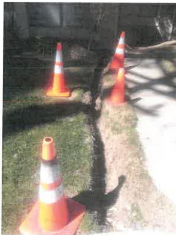
2015 - trench dug to remove drainage pipe clogged with tree roots causing rain water to accumulate on building roof.
