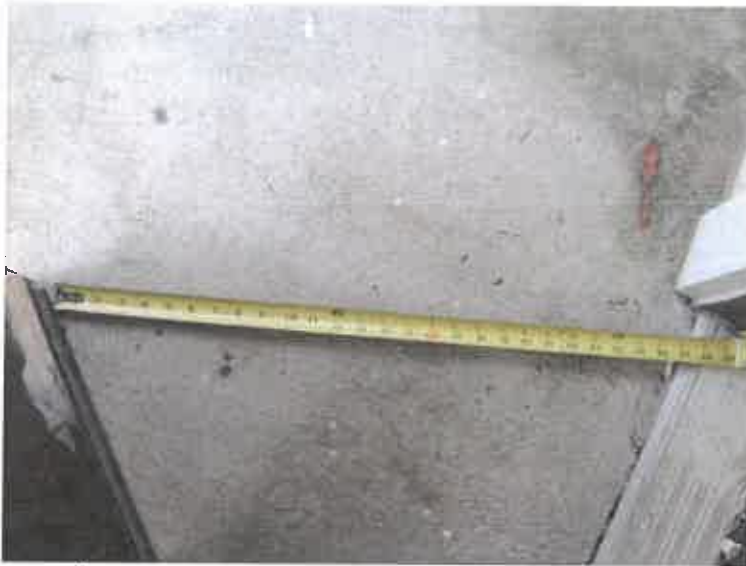
2007 - walkway at Suite 105 showing door opening to a maximum of 28 inches because of raised concrete caused by tree. To avoid this in the future, door was re-hung opening inward.
