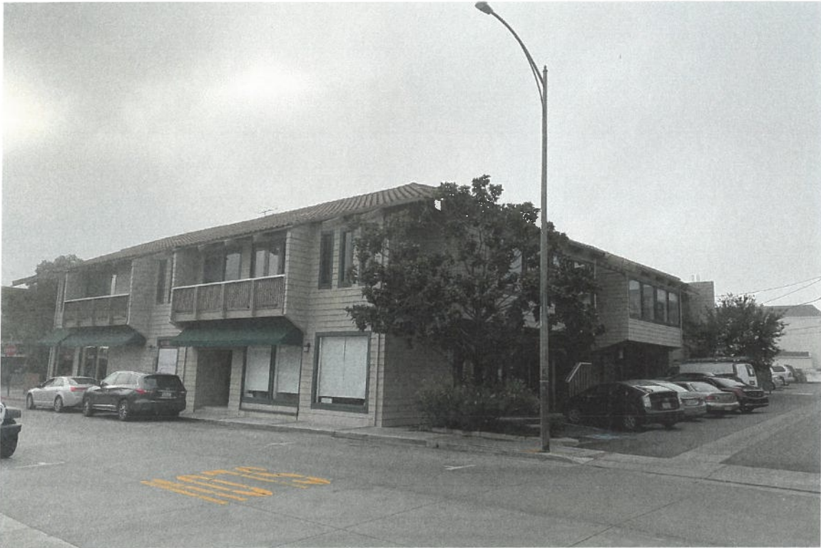
View #3 - Northwest Corner - Bean Ave & Victory Ln
