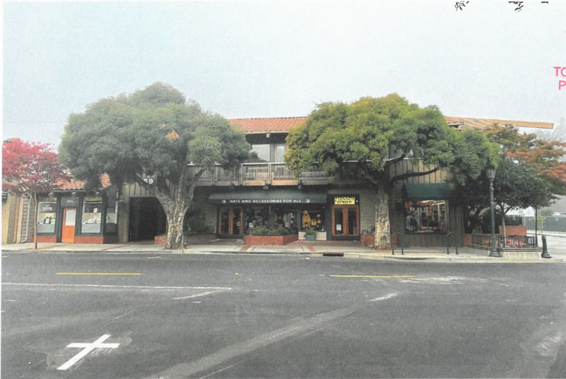
View #1 - East Elevation - N Santa Cruz Ave
