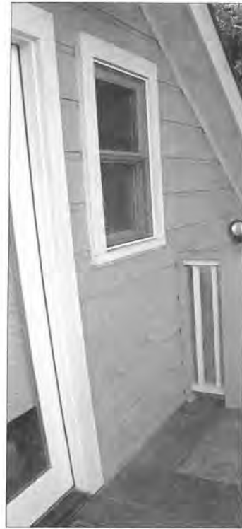
EXISTING WINDOW PHOTO
